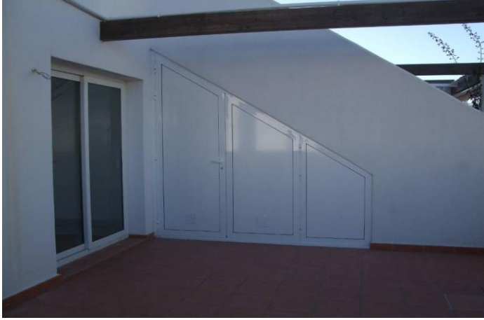
FIGURE 5.5A: STORAGE UNDER STAIRS
