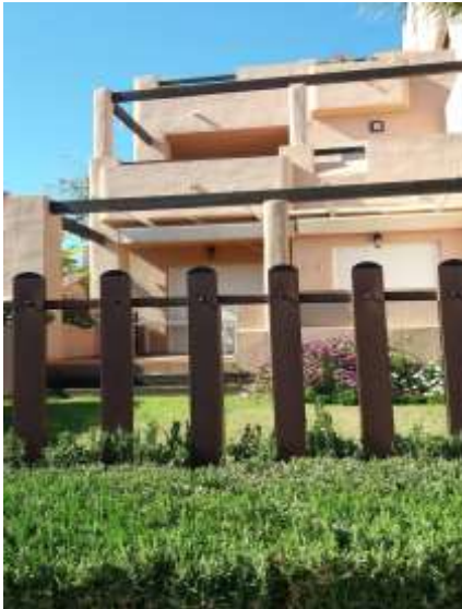
FIGURE 7.5: GROUND FLOOR FENCE
